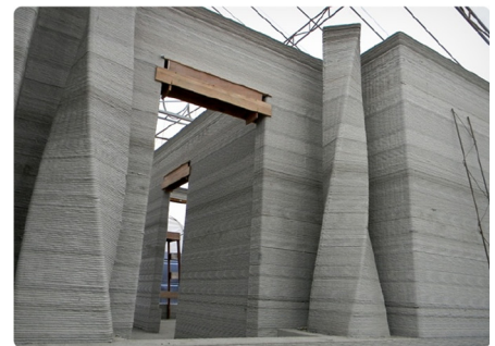
f) vertically printed, in-situ walls and columns. Image: courtesy of Andrey Rudenko, Total Kustom, USA
