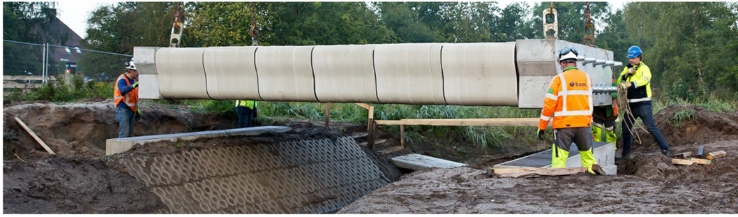
Fig. 8. The 3D concrete printed pedestrian and bicycle bridge in Gemert, the Netherlands, is hoisted into position.
