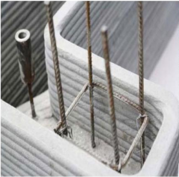
Fig. 9. Example of inclusion of passive reinforcement in a 3D printed concrete formwork (WinSun [33]).
