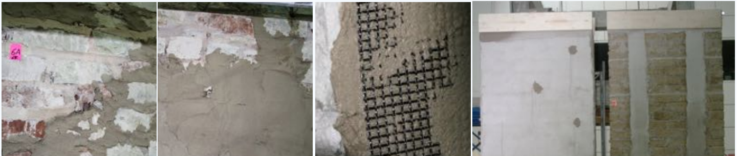
Textile Reinforced Mortar installation on the stone wall
