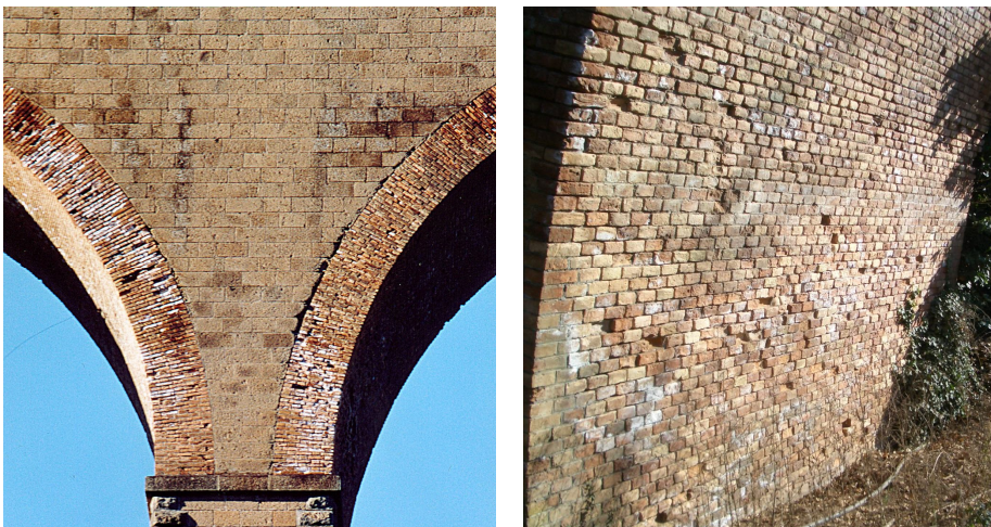
Figure 4.16. Vaults and spandrel walls (left) and detail of brick arrangement in the arches (right).
